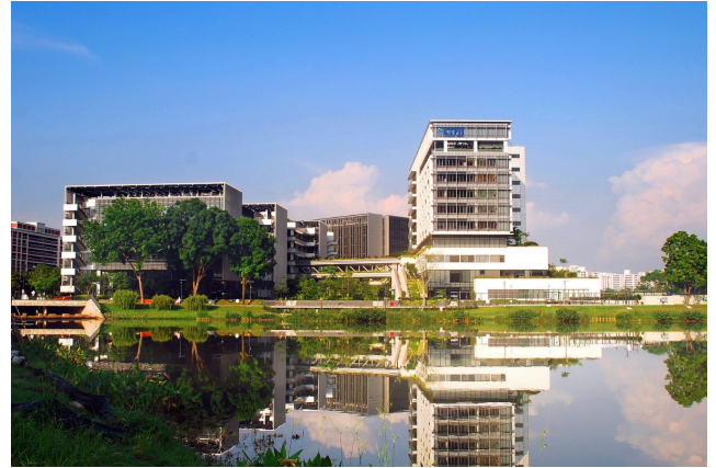
Рис.1.20 Viewed from across Yishun Pond, Khoo Teck Puat Hospital [56].
