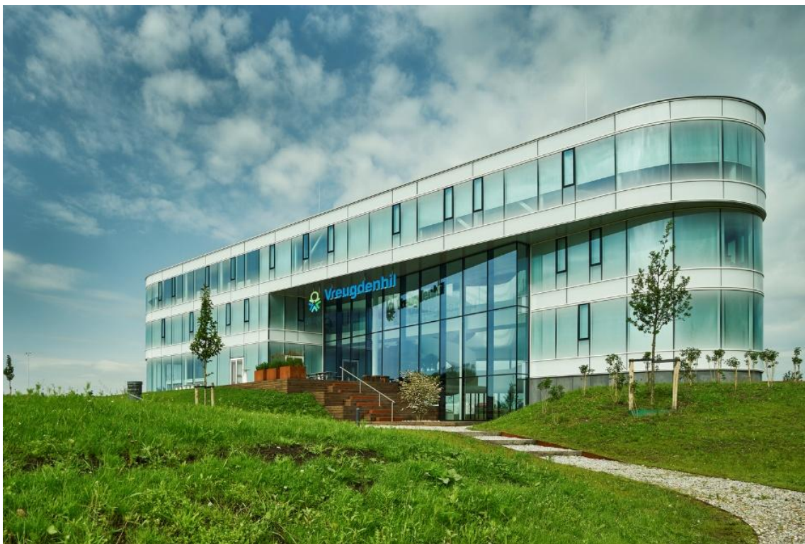
Рис. 2.5. Фасад New Highly-energy Efficient Office for Vreugdenhil[28]
