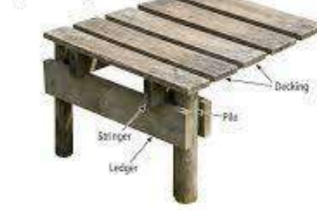
Boardwalk with sleepers
