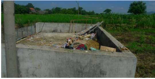
Current situation of garbage pool
