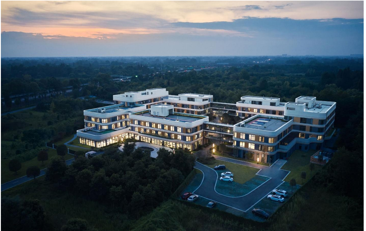
Рис. 2.6 CHUNTAIWANG Rehabilitation and Care Institution
