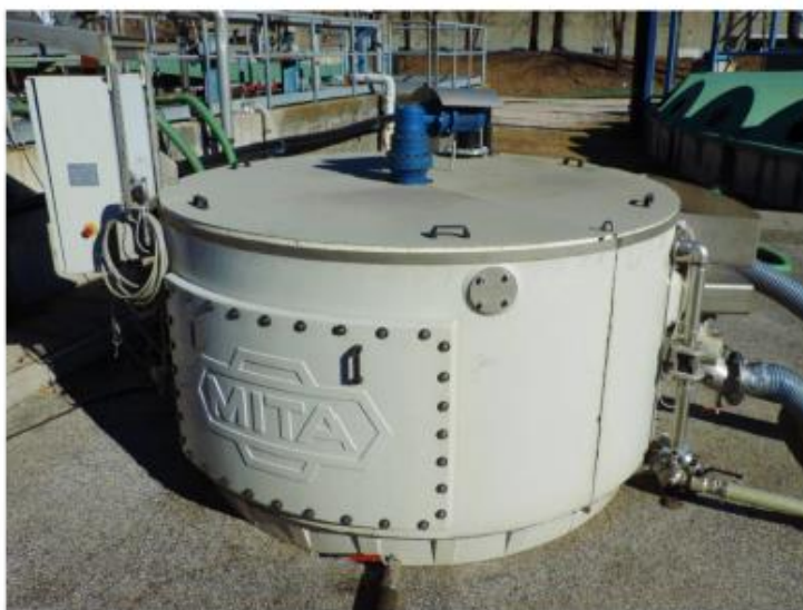
Figure 3. Photograph of the pilot cloth filtration plant installed in the studied wastewater treatment plant.
