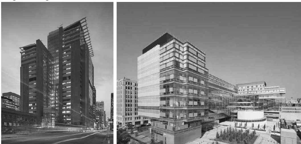
Calgary Courts Centre, Calgary, Canada [4].
