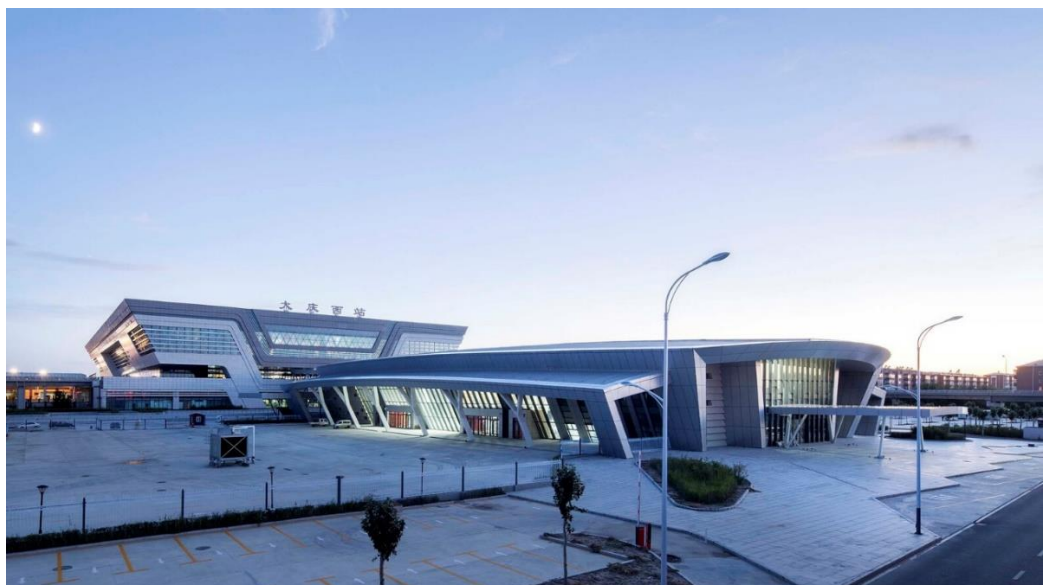
Рис. 1.15. Daqing West Integrated Highway Passenger Station
