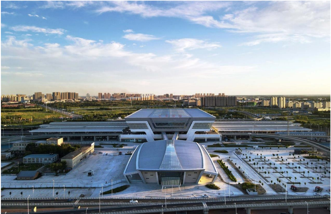
Рис. 1.14. Daqing West Integrated Highway Passenger Station
