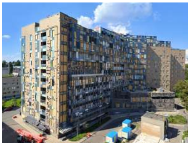
Figure 1. Exterior view of the inspected structure
