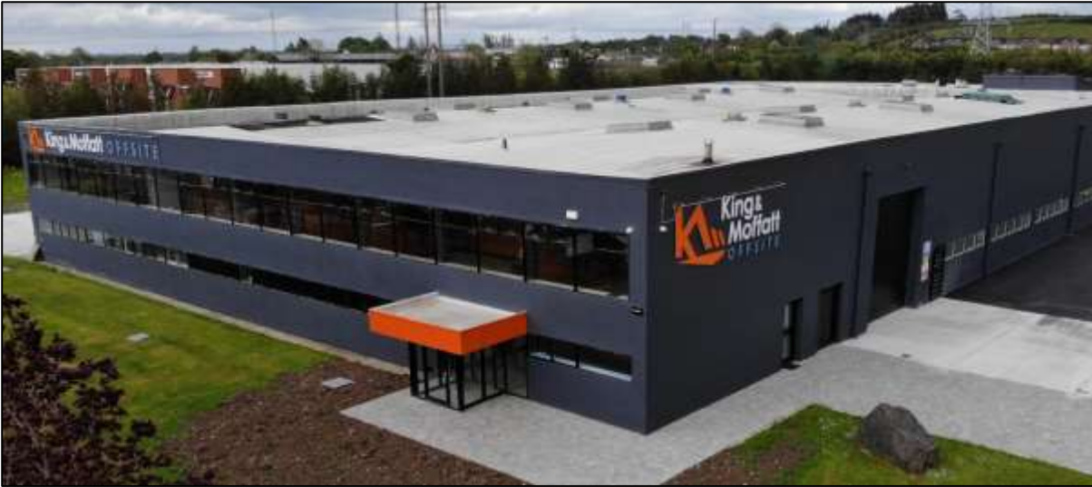
Figure 4: Prefabrication Precision: A Glimpse into King & Moffatt's Offsite MEP Facility
