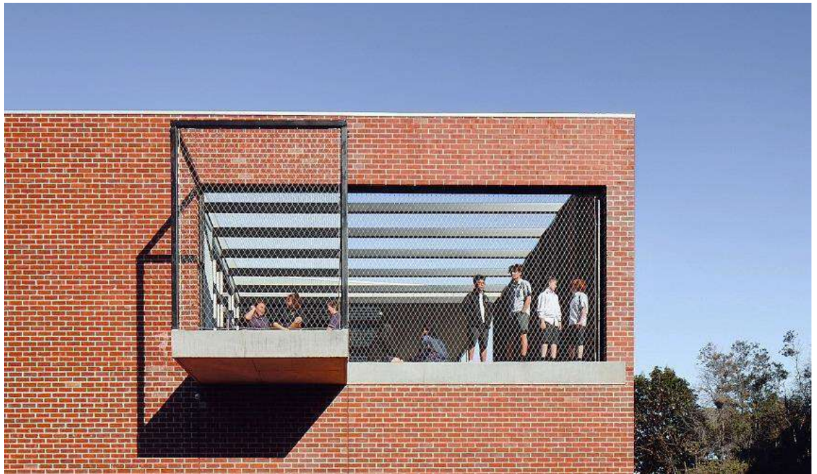
Рис. 1.3.7. Northcote High School Performing Arts & VCE Centre, Арх. КТА, Австралія
