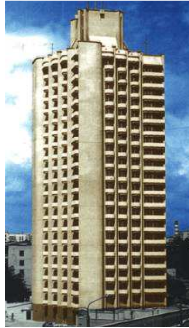
Fig. 9. The first residential house made without nay OPC from alkali- activated cement concrete (Lipetsk, Russian Federation)
