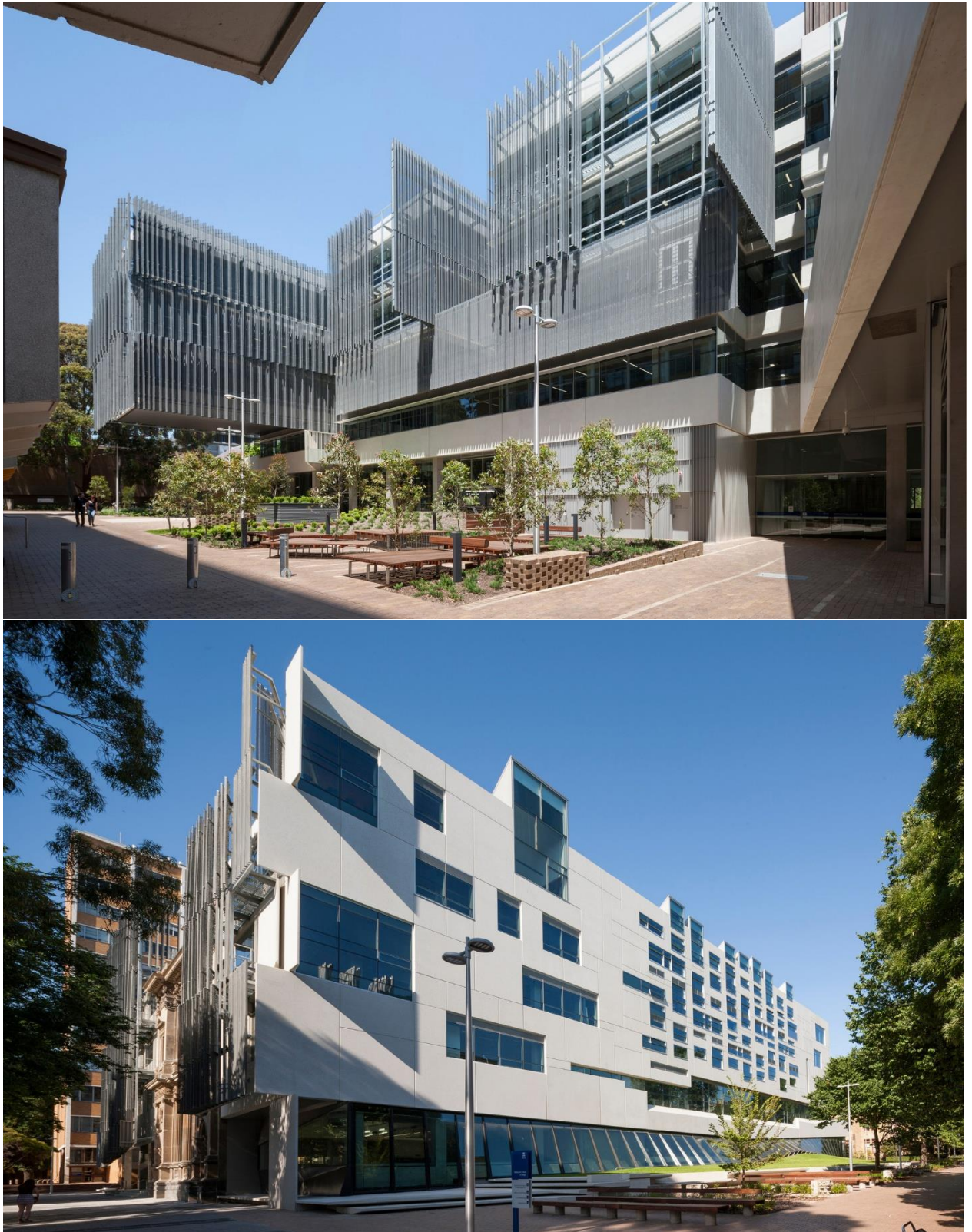
Рис.2.18. Melbourne School of Design University of Melbourne / NADAAA + John Wardle Architects [20]. Загальні вигляди.
