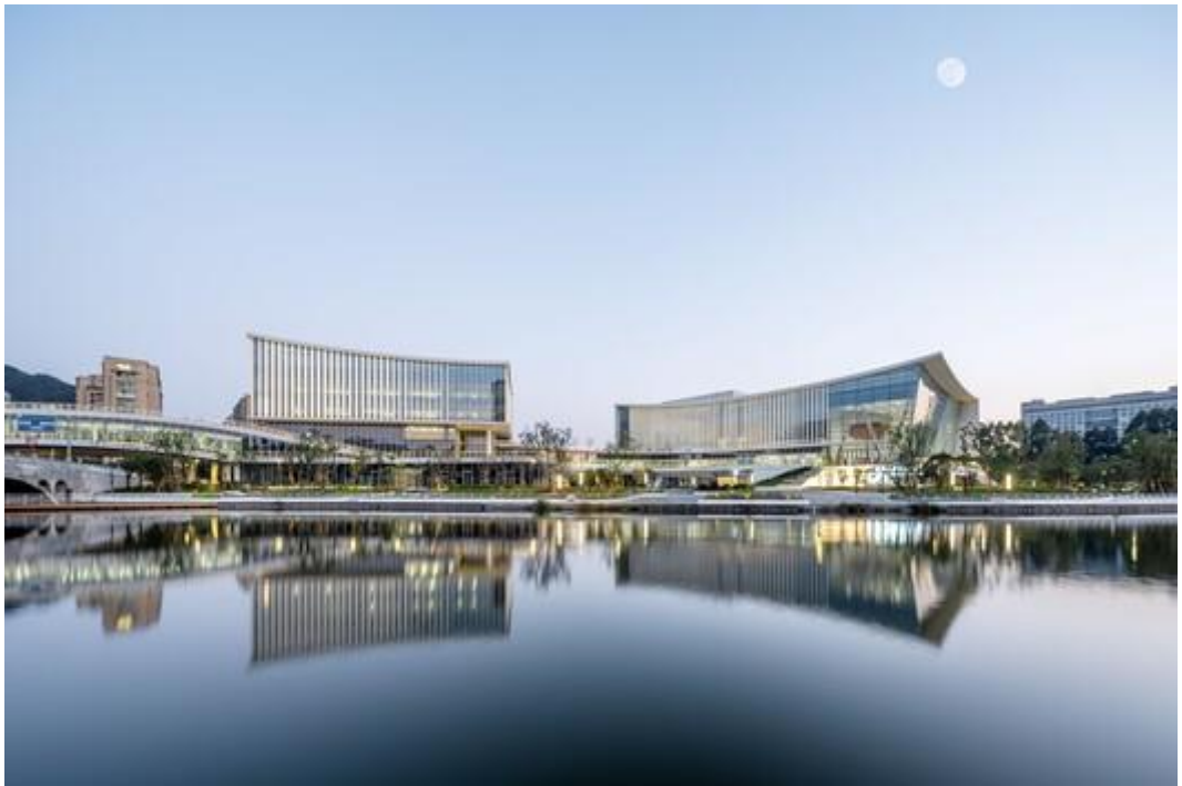
Рис.2.22. Фасад Wenzhou High-tech Cultural Square [13]
