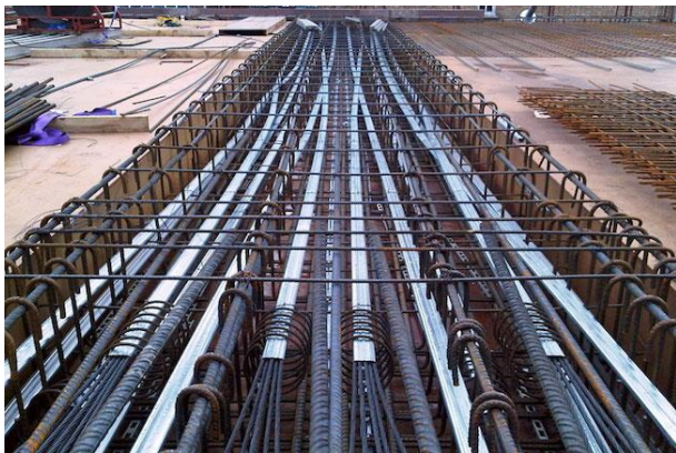
Figure 4. Using internal amplification «Internal Post-Tensioning»
