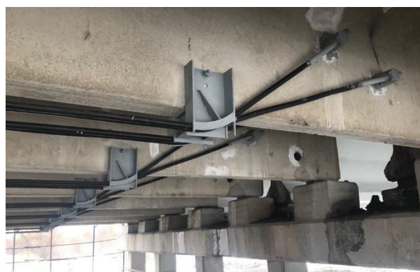
Figure 2. Use of external reinforcement "External Post-Tensioning"
