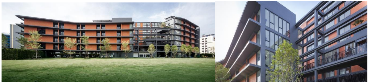
Рис. 1.16. Rose des Vents Student Housing. Фасад [29]
