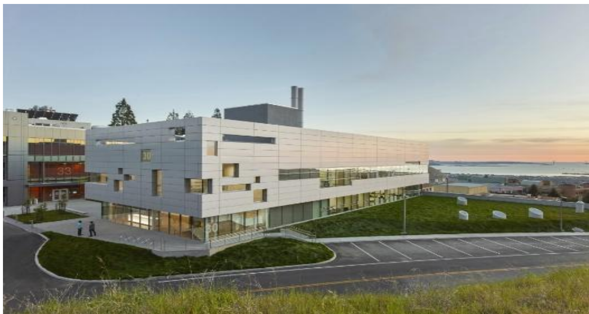
Рис. 2.6. “Chu Hall - Solar Energy Research Center” [6]
