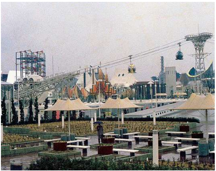
Fuji Pavilion, EXPO-70, Osaka, Japan
