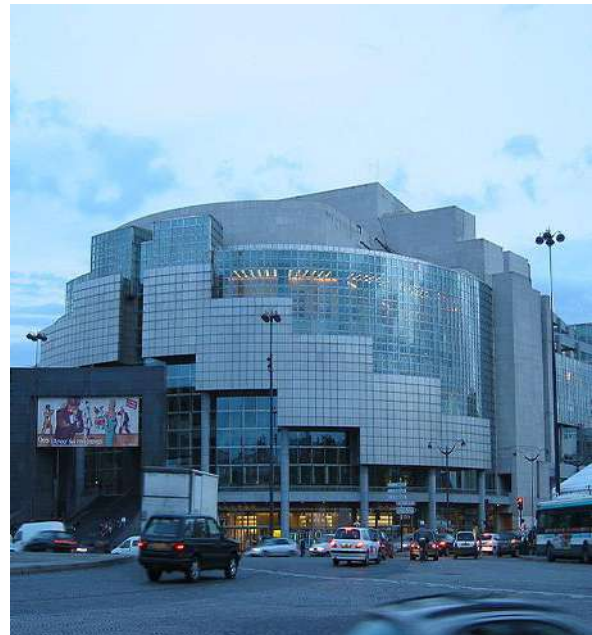
Opera de la Bastille, Paris, architect Carlos Ott, 1983-1989
