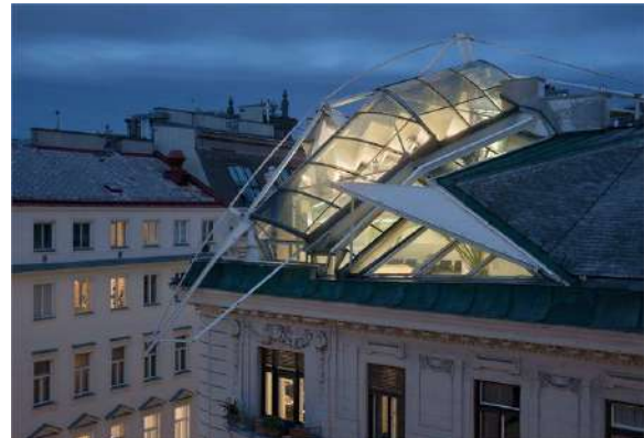
Reconstruction of the attic of a residential building, Vienna, Coop Himmelblau, 1988
