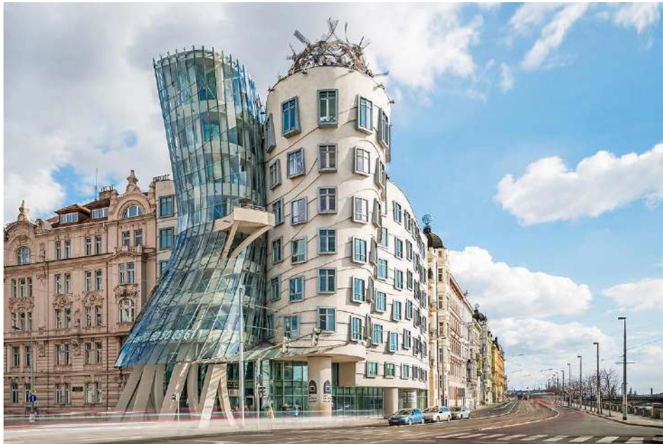
Residential building "Ginger and Fred", Prague, architect F. Gehry, 1996
