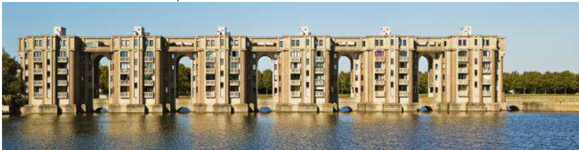
Residential complex "Lake arcades", France, architect Ricardo Bofill, 1982
