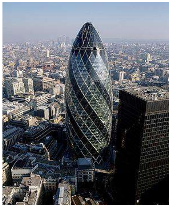
Office building "30 St Mary Ax", London, architect Norman Foster
