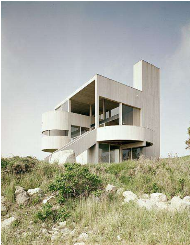
Cooper Residence, Orleans, architect Michael Graves, 1968-1969
