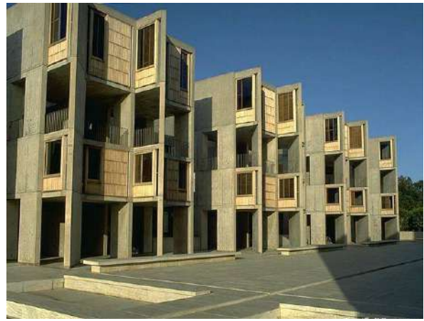
Salk Institute Research Center, California, architect Louis Kahn, 1966
