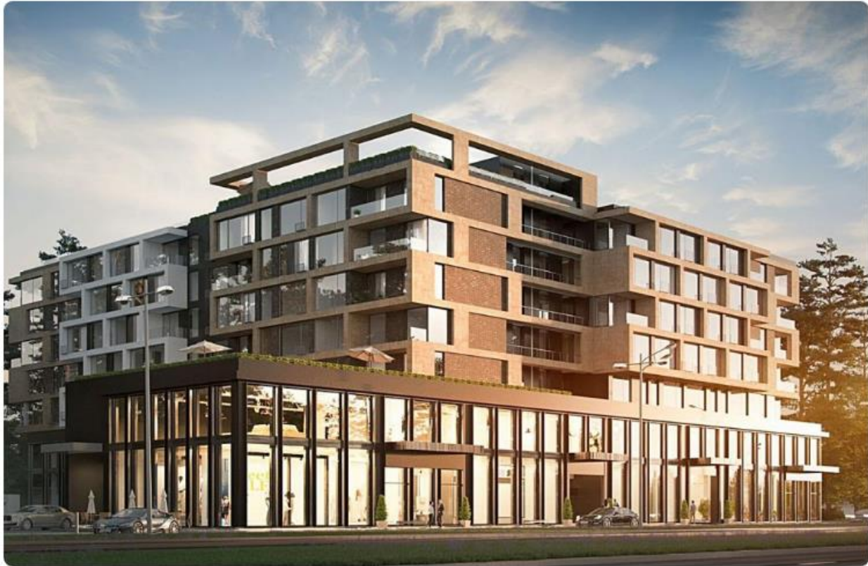
Fig. 2.5. View of residential complex "Pushcha House"
