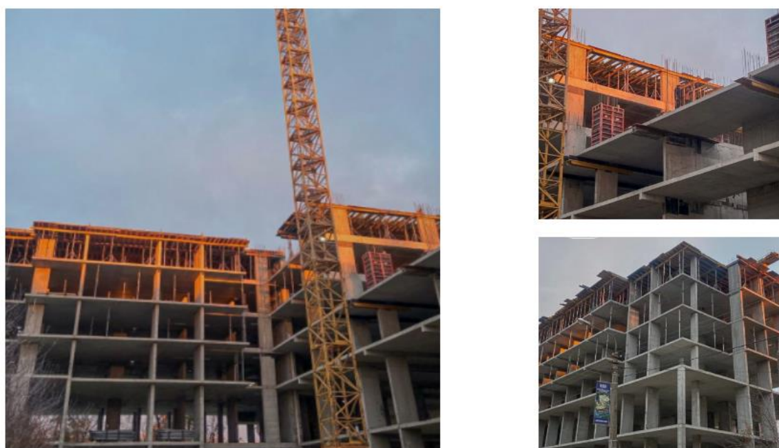
Fig. 2.13. Construction progress of the PushaHouse apartment building
