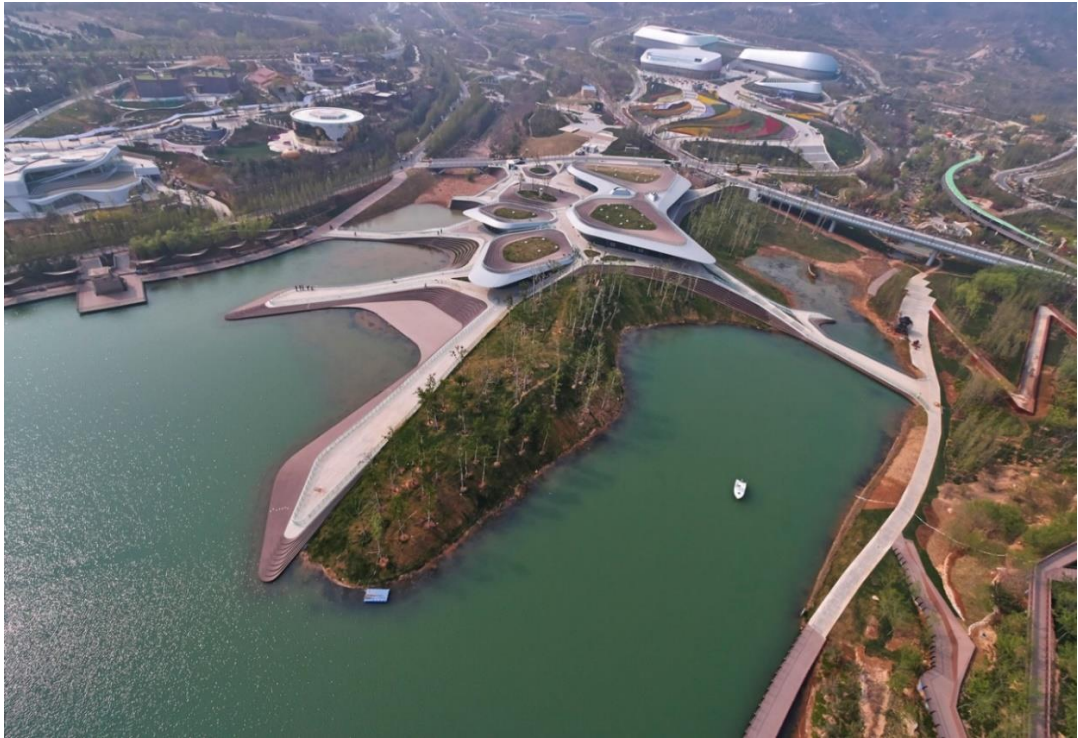
Рис.2.6. Heavenly Water Service Center of International Horticultural Exposition[4]
