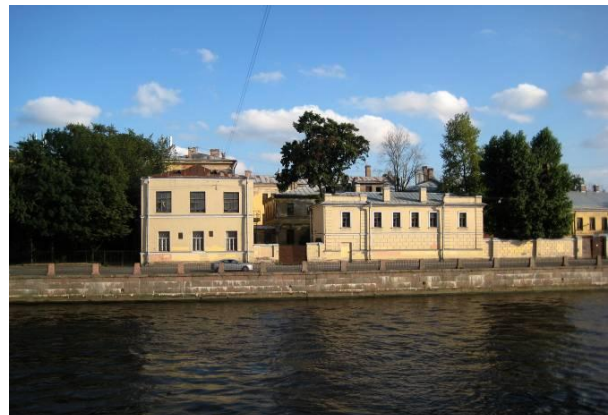
Figure 18. Alexander Hospital. St. Petersburg
