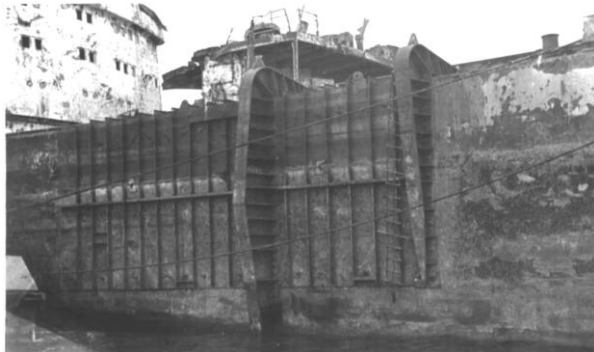
Fig.8. The path (7×14 m) welded with semi-automatic welding
