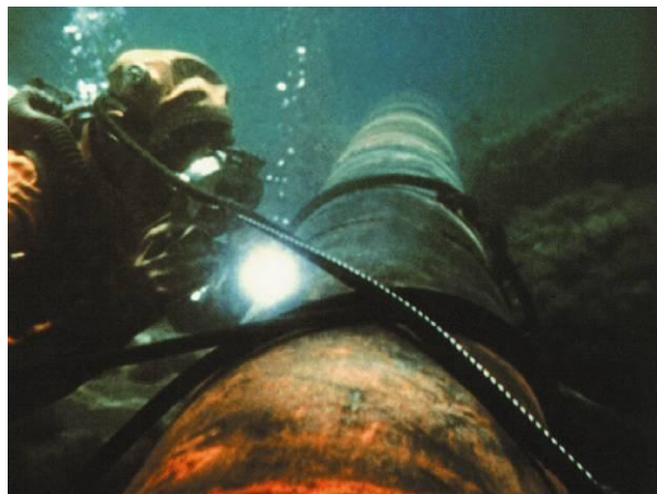
Fig.6. Wet semi-automatic welding of pipeline
